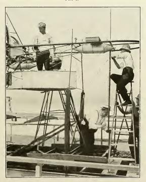
${\bf Fig.}\ \ 2.$   ${\bf GUY\text{-}POST}\ {\bf AND}\ {\bf PIN}\ {\bf ON}\ {\bf LAUNCHING}\ {\bf CAR}$
